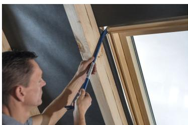
If the sash is not parallel with the frame, you can use a crowbar to set the gap.
