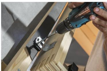
If the vertical gap is not parallel, use the black plastic wedge for the top brackets. If the frame is correctly aligned, fix the top brackets (and side brackets if exist) as well.
