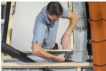
When fixing the side pieces, make sure you cut and tightly secure around roof battens.
