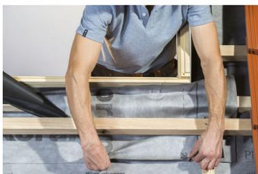
Loosen the batten underneath the frame to allow for the positioning of the membrane.
