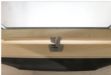
Check if the horizontal gap is parallel at the bottom when in a slightly opened position.
